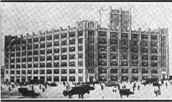
New eight-story factory of the American Ever Ready Co., Long Island City, N. Y., 200 by 300 feet and representing an expenditure of $1,000,000
